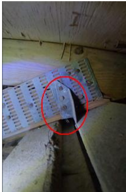
Roof to Wall Attachment (clip)
