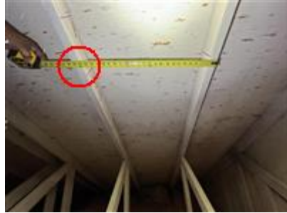
Truss Spacing (24" OC)
