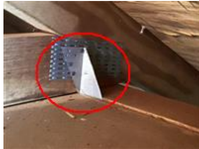
Roof to Wall Attachment (Clip)
