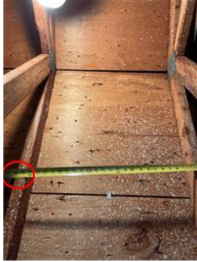
Truss Spacing (24" OC)
