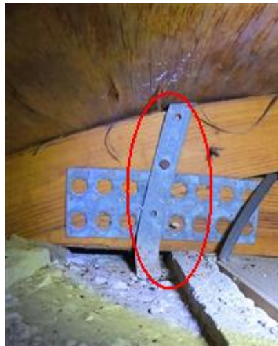
Roof to Wall Attachment
