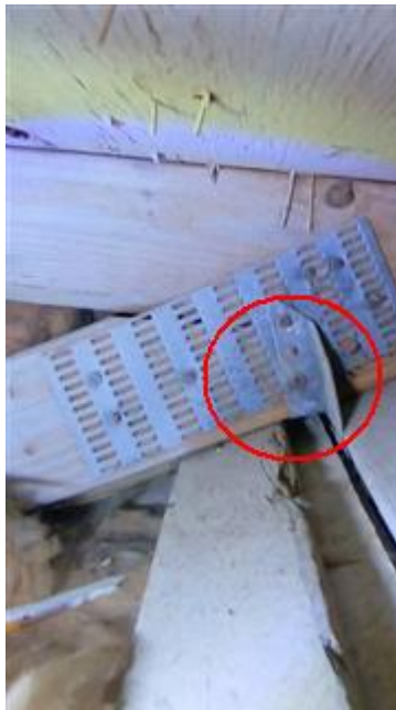
Roof to Wall Attachment (Clip)
