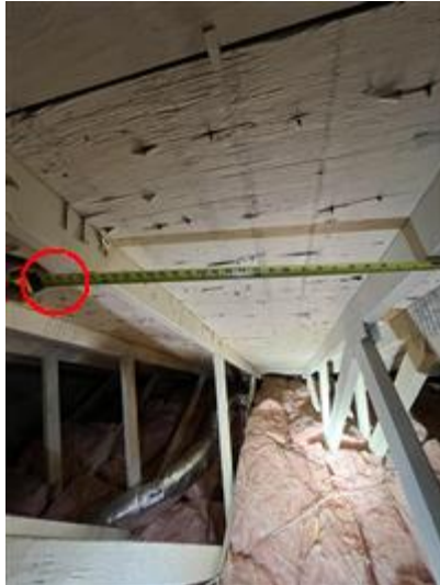
Truss Spacing (24" OC)
