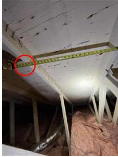
Truss Spacing (24" OC)
